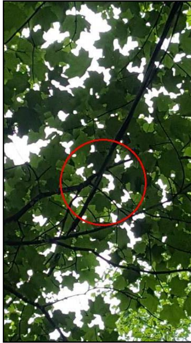
6. Branches, vines interfering with wires
