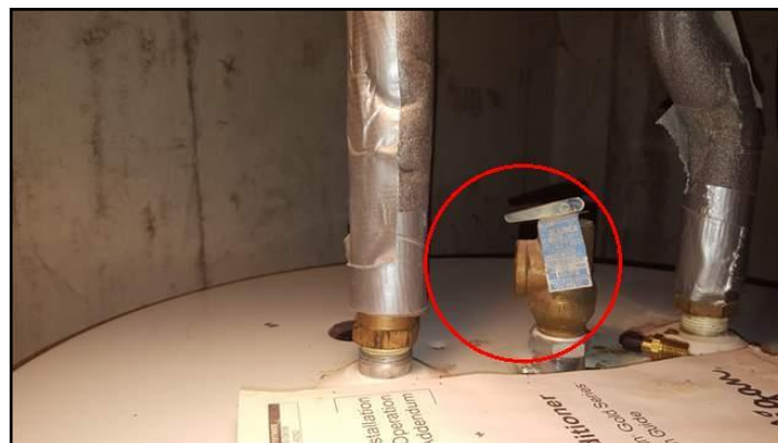
21. Discharge tube missing
