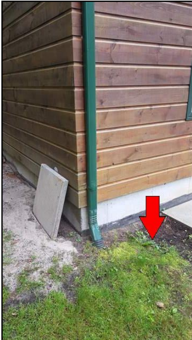
1. Downspouts discharging below grade
