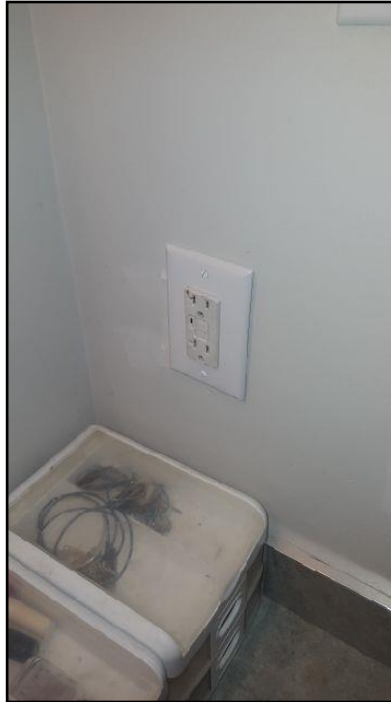
14. Test faulty on GFCI/GFI (Ground Fault...
