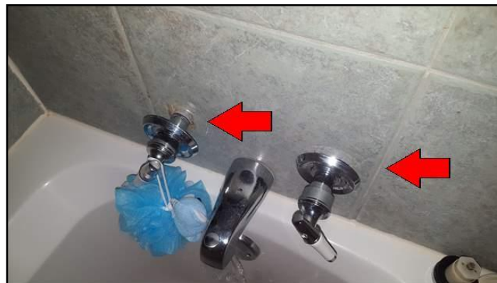
25. Caulking loose, missing or deteriorated
