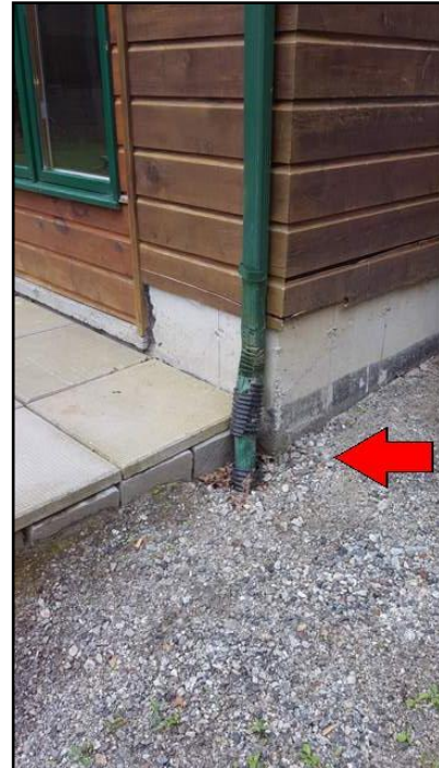
2. Downspouts discharging below grade
