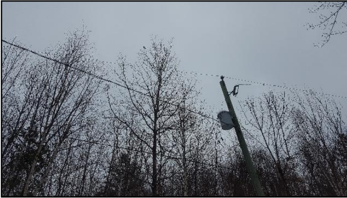
23. Branches / vines interfering with wires
