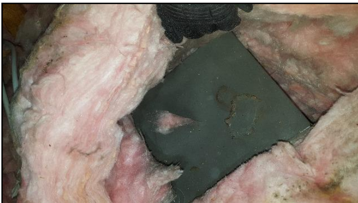
44. Poor termination location
