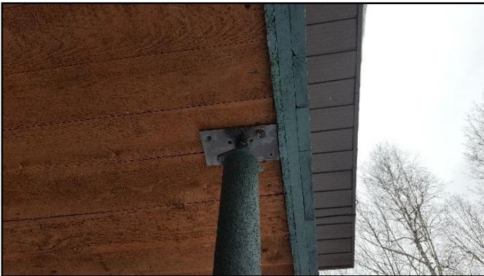
19. Poorly secured at top
