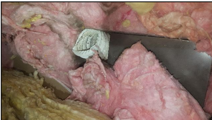
42. Poor termination location
