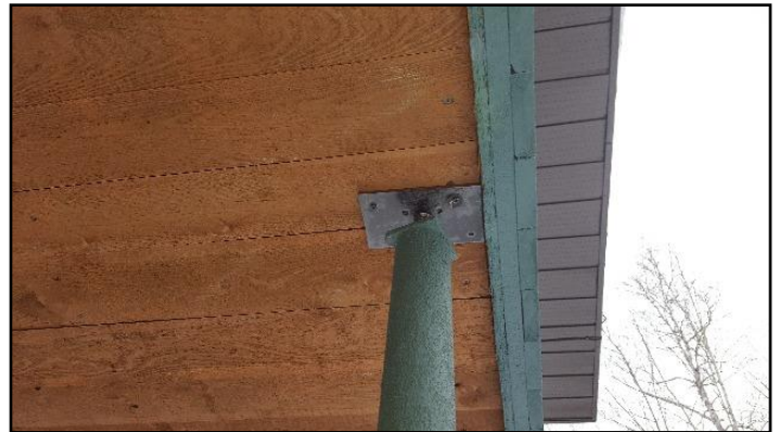
20. Poorly secured at top
