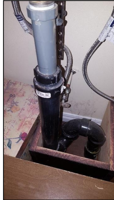
48. Nonstandard shape or material
