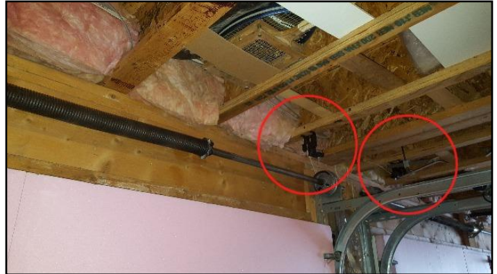
16. Sensors poorly located
