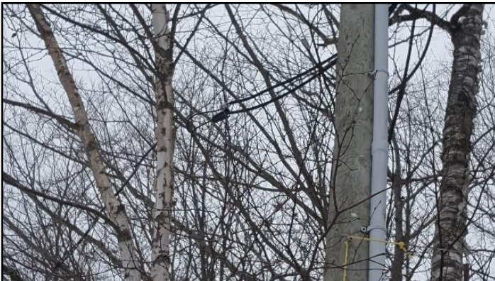
21. Branches / vines interfering with wires
