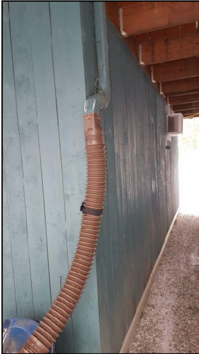
4. Should discharge 6 feet from building
