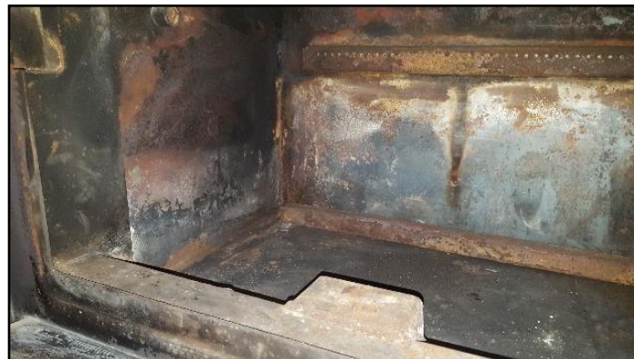
37. Firebrick missing
