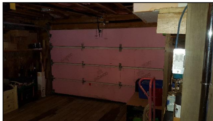
13. Combustible insulation
