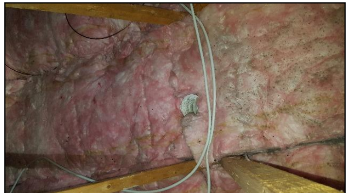
43. Poor termination location
