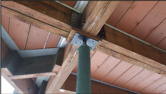
17. Poorly secured at top
