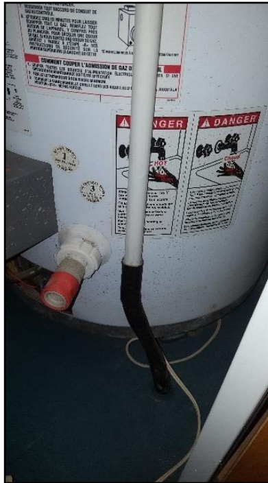
46. Discharge tube capped
