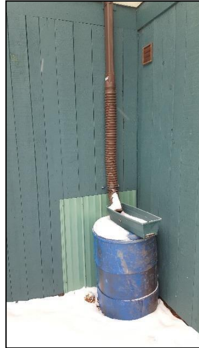
5. Should discharge 6 feet from building
