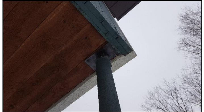
18. Poorly secured at top
