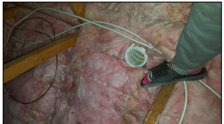
45. Poor termination location
