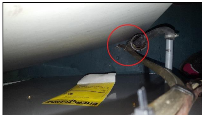
38. Improper discharge point
